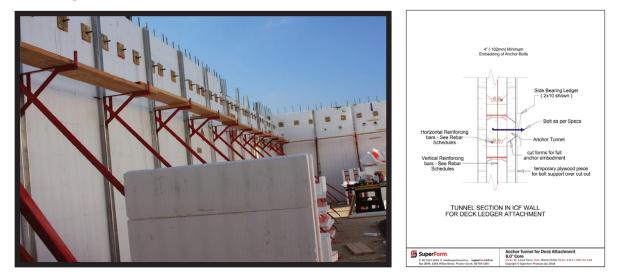
**Concrete floor:** The exterior ICF panel should continue through with the interior one being cut off the thickness of the floor. There are numerous types of concrete floor systems. All systems must bear on the concrete.
