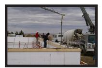
Consolidation is the removal of entrapped air in the concrete. Because the EPS does not come off you need to be sure that there are no voids in the wall. Consolidation ensures that the rebar is properly embedded in the concrete.
