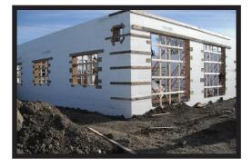
Blocks may need to be cut horizontally above or below openings. Using a skill saw works good for this.
