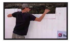
For sake of efficiency always try to only cut blocks either on the top or bottom of your opening. If you cut the bottom row of ICF the top row should run over the window buck. If you cut the block above the window buck the buck should sit on the 4th/5th row etc.
