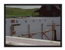
Run string lines to make sure your wall is straight. The string line is typically run on the opposite side of bracing. Use the stringline to adjust walls before and after pour. **Before placing concrete ensure the walls are slightly tilted in.** It's a lot easier to push the wall out then pull it in with the weight of the concrete in it.
